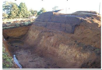
Over the next few weeks the geogrid exposed on the front face of the restored embankment will be covered with instant turf to prevent erosion, stop the geogrid deteriorating from UV exposure, and generally give the section of wall a finished look from the street. In the next stage of the restoration work the use of sandbags rather than formwork will be trialled as well as putting instant turf inside the geogrid rather than on top of it.
